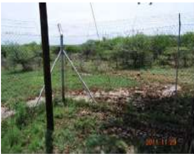
Sludge flowing out of plant
