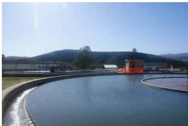
Figure 3: Loerie Water Treatment Works
