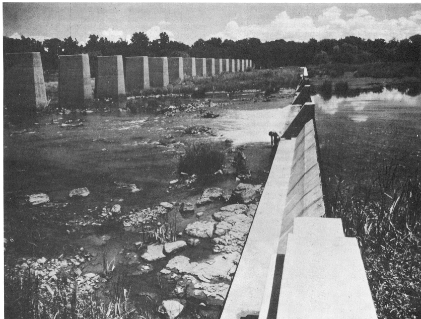
Meetdam in die Vaalrivier by De Hoop. Oor die 700 meetstasies in die vernaamste riviere in Suid-Afrika word deur die Afdeling Hidrologie beheer. Gauging weir in the Vaal River at De Hoop. More than 700 gauging stations in the most important rivers in South Africa are operated by the Division of Hydrology.
