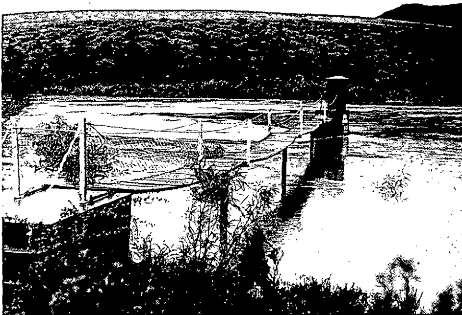
Fig. 6.6 Drie Heuwels Weir during Winter flood flow, note total submergence of weir.
