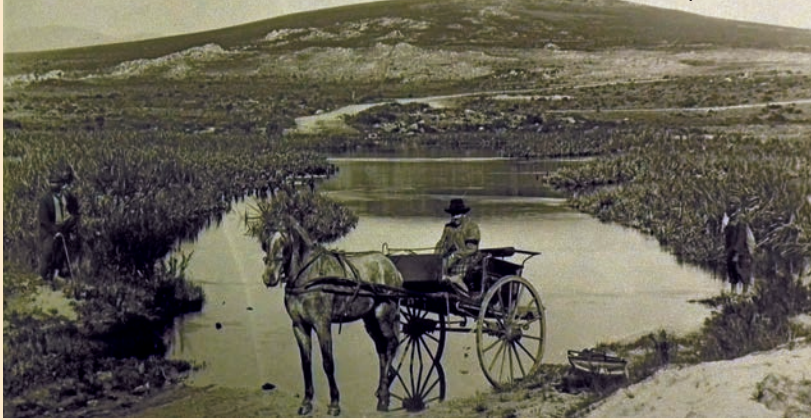
Grabouw Road over the Riviersonderend River near Villiersdorp
