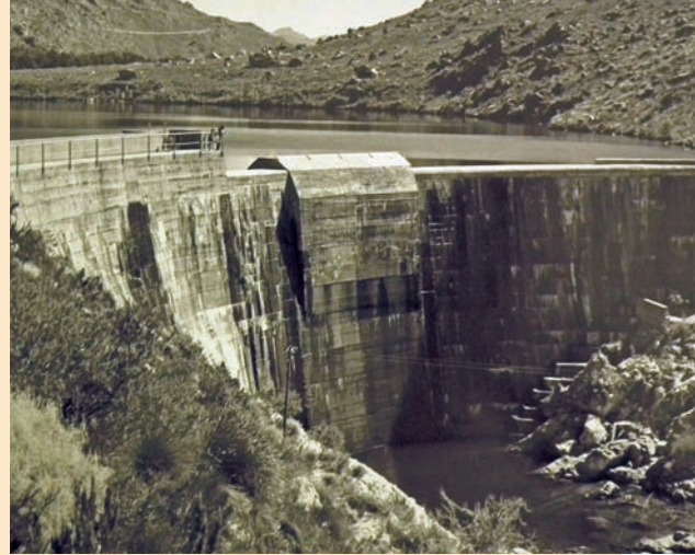
Ceres Dam in the Koekedouw River in 1977
