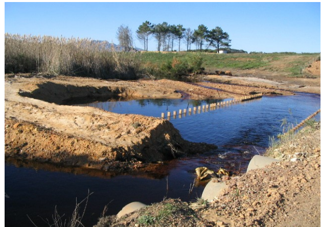
Plate 18. Site 3 Uilkraal River after construction – May 2005 (upstream)
