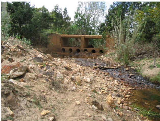
Plate 3. Site B2 – October 2004 (looking upstream)
