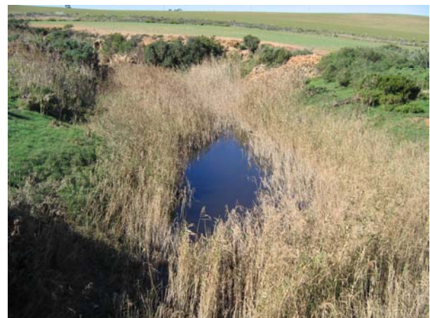
Plate 34. DWAF weir – October 2004 (looking downstream)
