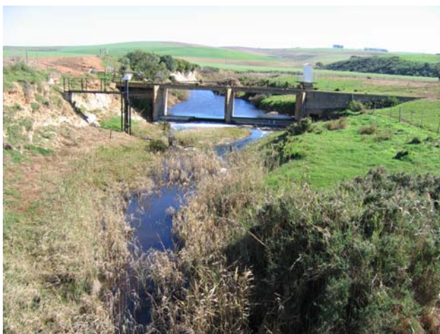
Plate 33. DWAF weir – October 2004 (looking upstream)
