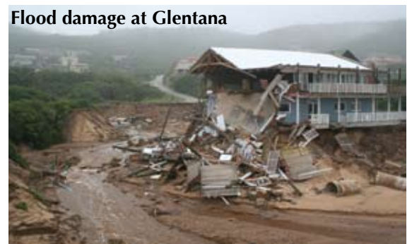
Flood damage at Glentana
