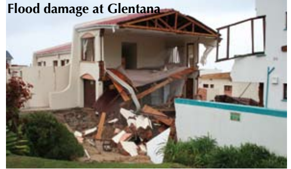
Flood damage at Glentana
