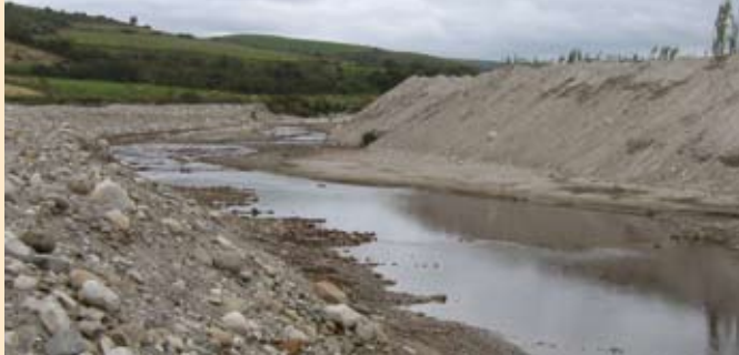
Channel modification in the Duiwenhoks River
