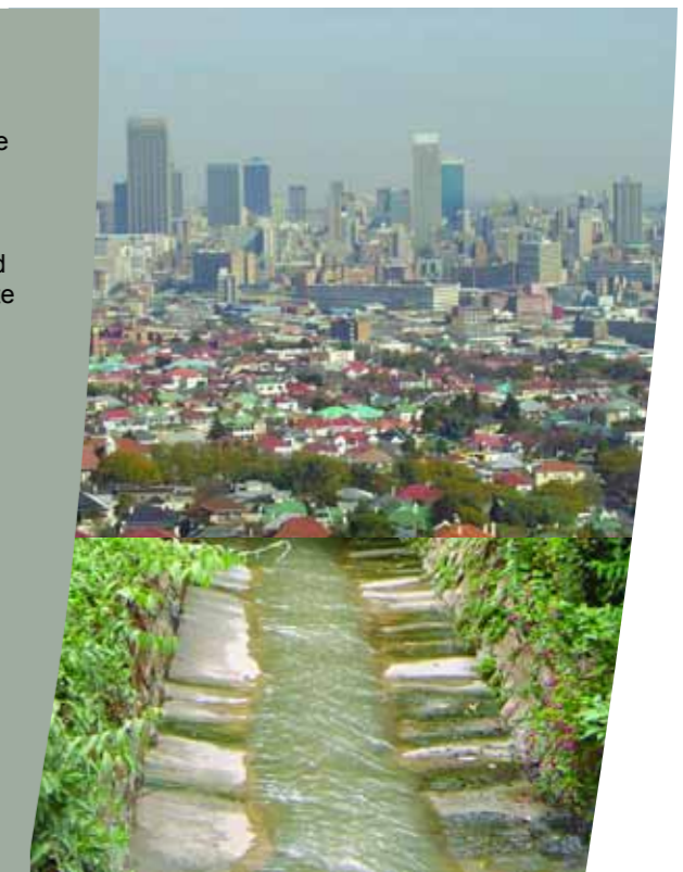
Johannesburg Canalised stream running through Johannesburg
