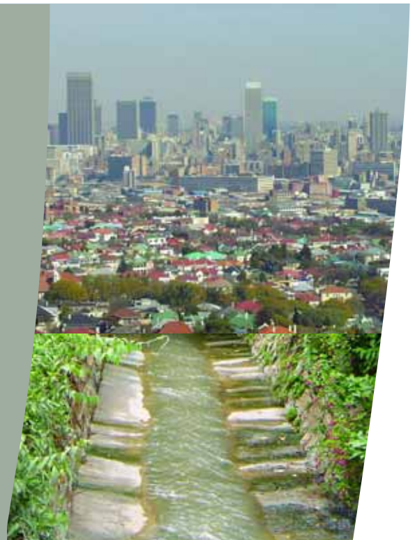
Johannesburg Canalised stream running through Johannesburg
