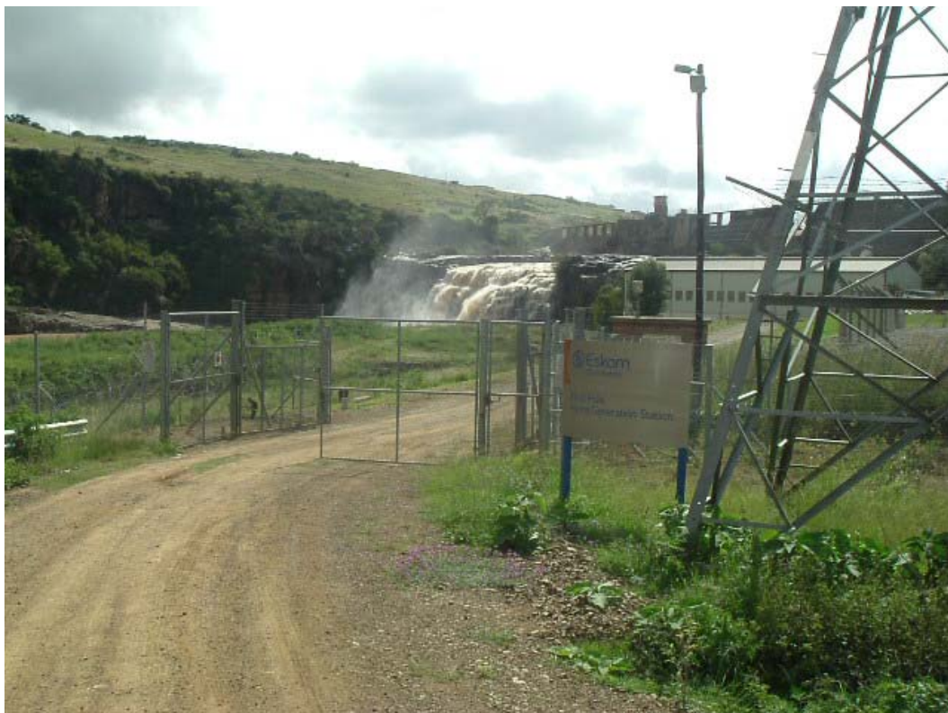
Plate 2.2 Hydropower plant at First Falls Dam on the Mthatha River
