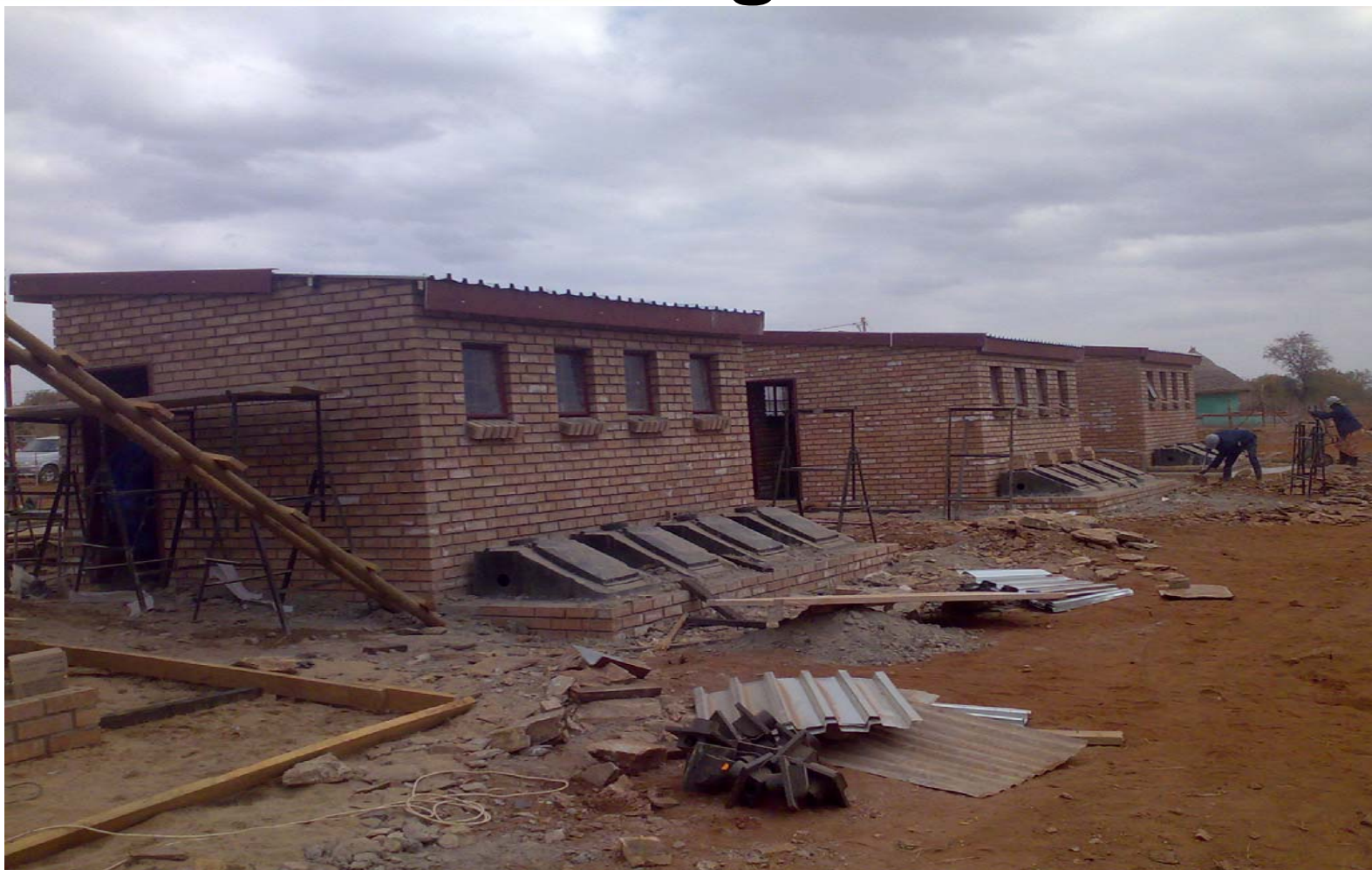
Muyexe primary school sanitation project 14/08/2009
