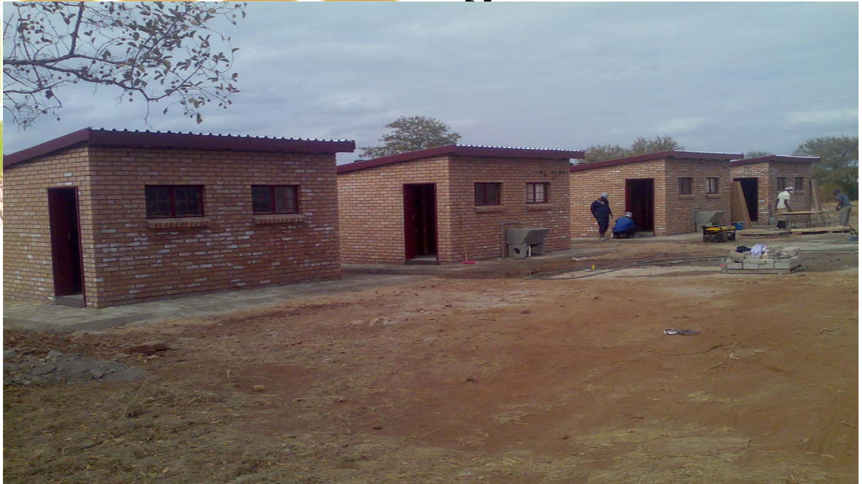
Hatlani Muyexe high school sanitation project 14/08/2009
